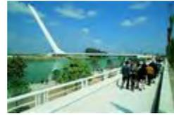
Cantilever spar cable-stayed bridge
