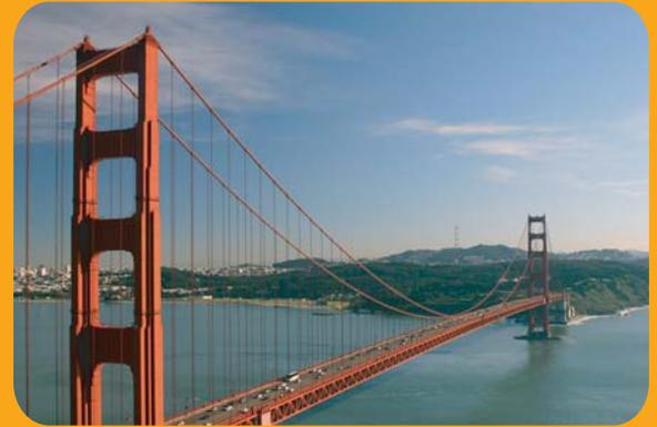
The suspension bridge is the most often used design for long bridges. When it opened in 1937, the Golden Gate Bridge was the longest suspension bridge in the world. It quickly became the symbol of the city of San Francisco and today it is one of the most photographed bridges ever. Why is the bridge painted in orange? The color makes it visible in fog.
