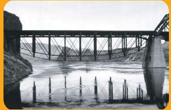
Trusses are made of small elements connected in triangles. When you place the weight on the deck, the truss wants to bend down and pushes on the rope. The rope wants to stretch so it pushes the deck blocks in. This makes the truss rigid and strong. In general, trusses use less material but take more space than solid beams of the same strength. Can you see this in the Burlington Northern Railroad in Schwana, WA?
