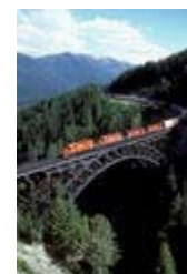
Truss arch bridge
