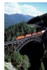
Truss arch bridge
