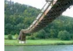
Stressed ribbon bridge
