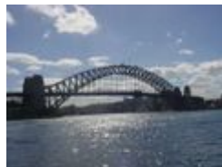
Compression arch suspended-deck bridge
