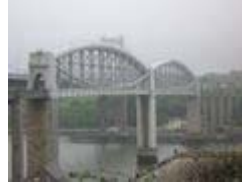
Brunel Truss bridge or lenticular truss
