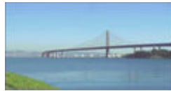
Self-anchored suspension bridge
