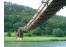
Stressed ribbon bridge
