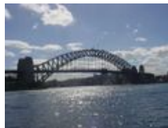
Compression arch suspended-deck bridge
