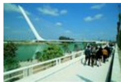
Cantilever spar cable-stayed bridge
