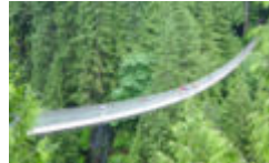
Simple suspension bridge
