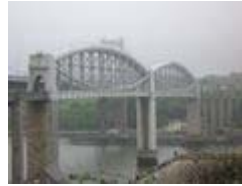
Brunel Truss bridge or lenticular truss
